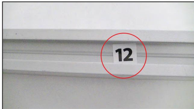
Detail B: Each extrusion contains a numbered label that corresponds to set-up instructions. The label is located within a groove of the extrusion (when possible). The numbers are black unless otherwise specified.
